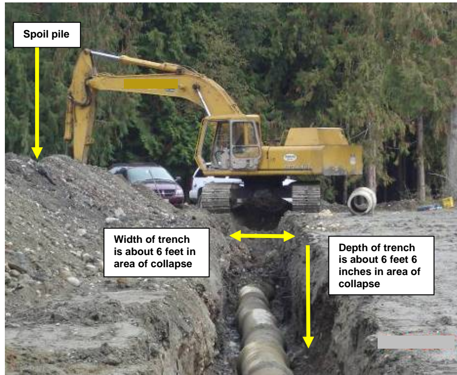
Figure 1: The excavator used to dig the trench.
